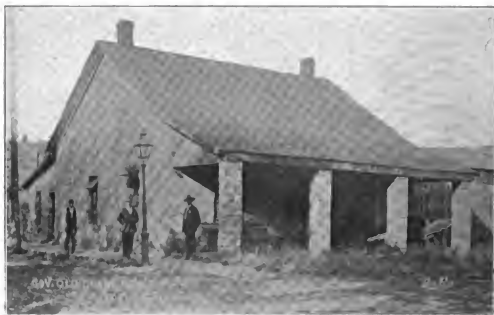
OLD GUARD HOUSE, FORT SCOTT.
